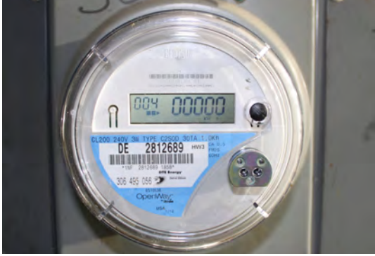
A residential electricity meter. Photo by Dwight Burdette . CC-BY-3.0.
